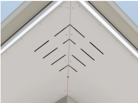
Step 7. Fix the 2nd mitered sheet according to design table and sheet edge fastening recommendations. Then scrape off excess epoxy.
