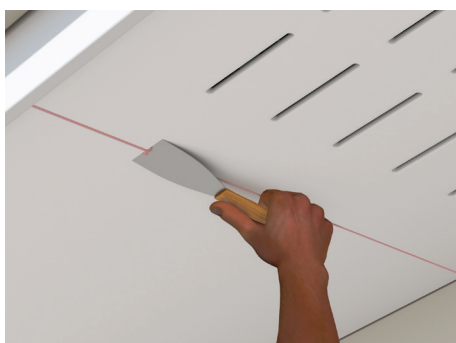
Step 5. Scrape free the excess epoxy to avoid bulge spots on the joint.
