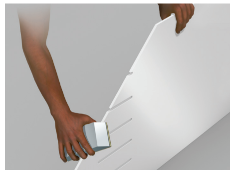
Step 3. Cut out the excess piece and clean edges with sandpaper.
