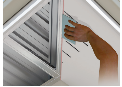
Step 6. Butter the edge of the 1st sheet with a thin layer of the epoxy. Take note to mix only a small amount of Epoxy to avoid wastage due to premature hardening.
