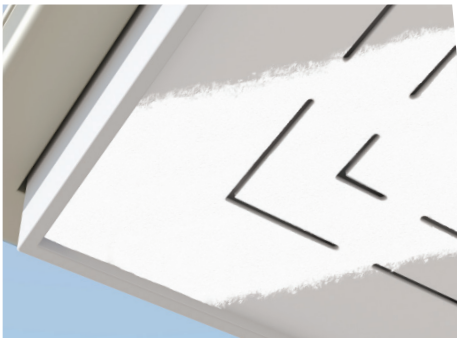
Step 5. Apply succeeding coats of HardiePutty™ until mesh tape is fully covered. Carefully feather out the edges with a minimum spread coat of 250mm wide. Clean excess HardiePutty™ before applying.
